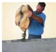
Loose fill is hard to handle and blows away easily in the breeze.
