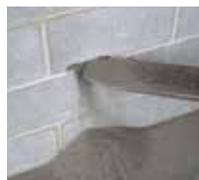
Loose fill drains out of the wall if puncture occurs, with no way to reinstall it.
