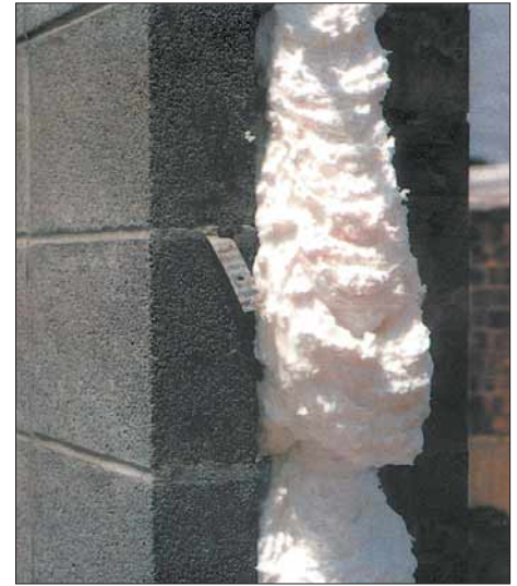
Polymaster R-501 applied in wythe cavity
