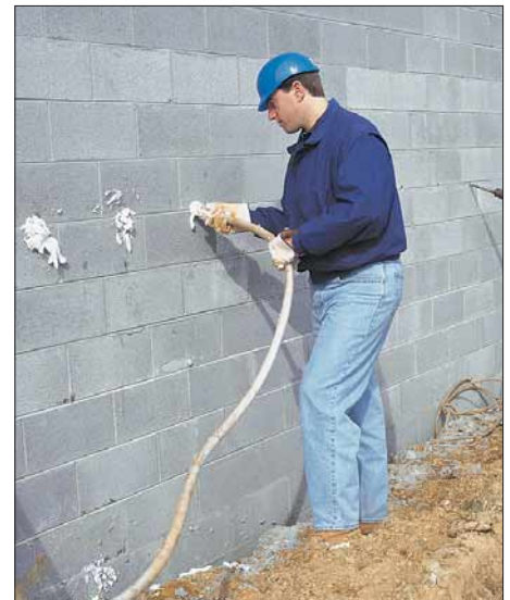
Typical installation technique for Polymaster R-501
